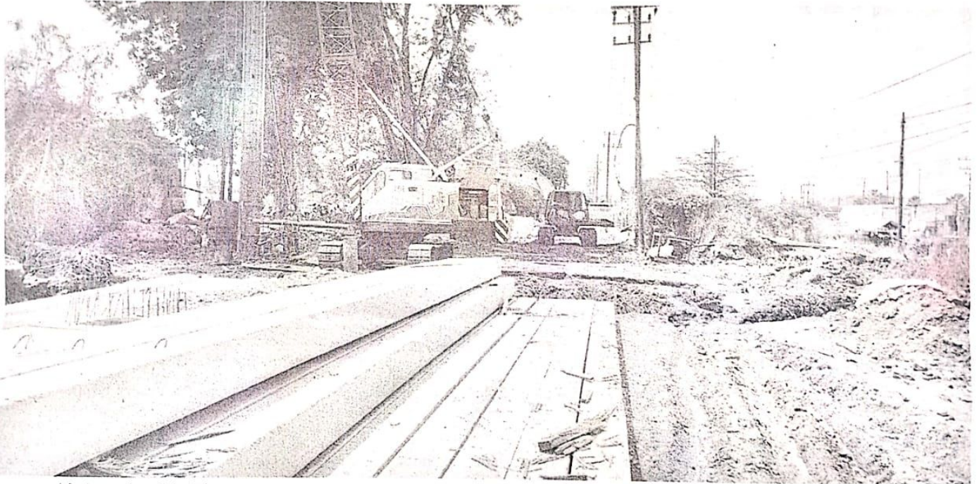
Progres proyek frontage road ruas Delta Sari.
